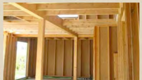
Construction ossature bois
